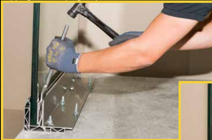
Tapping the clamping strip
