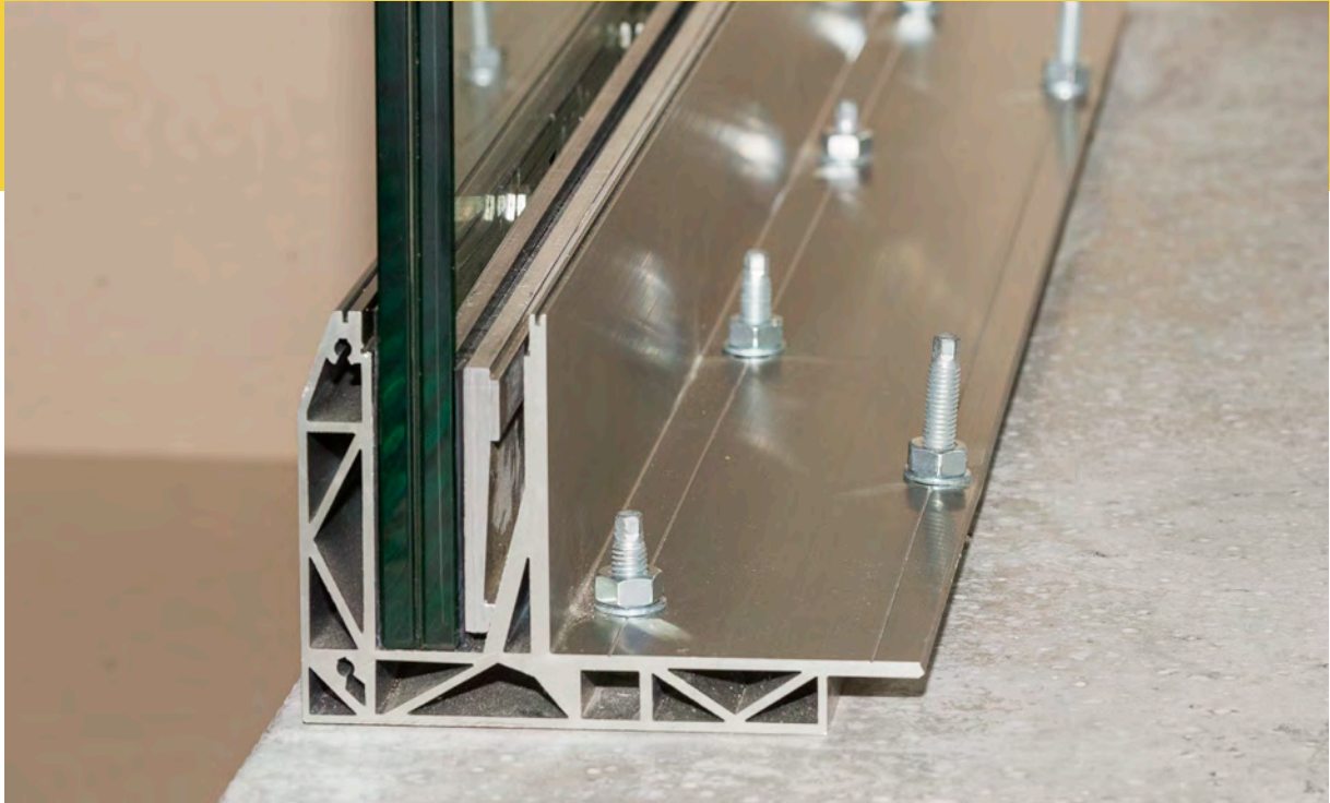
The continuous clamping strip is clearly visible
