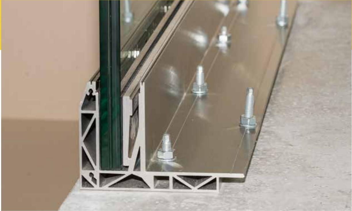
The continuous clamping strip is clearly visible
